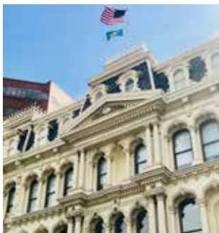
Window restoration - after
